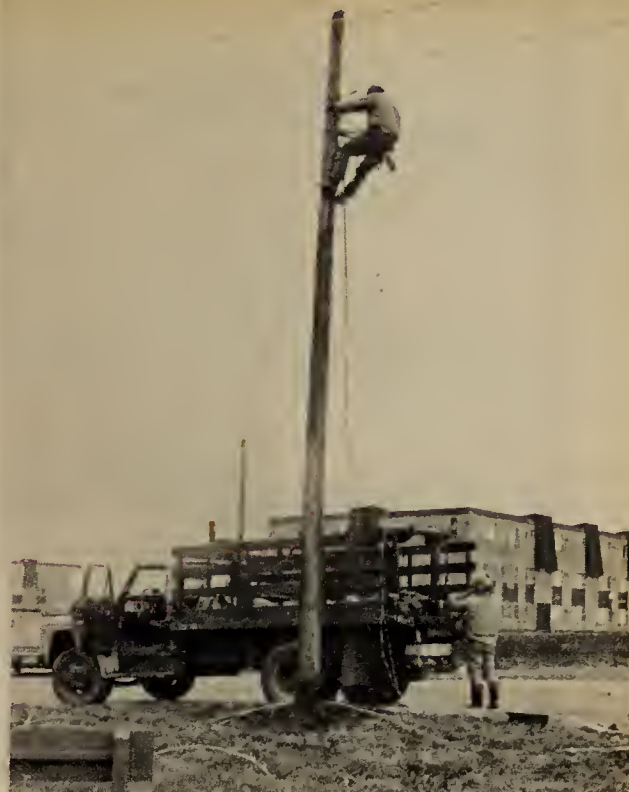
Workmen at Lambert and North Campus Rds. installing poles Nov. 27 to hold temporary traffic lights. — Photo by Scott Burket.
