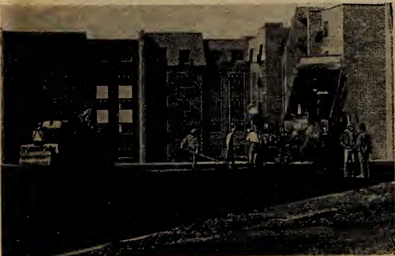
Workmen spread asphalt as construction on A building parking lots and North Lambert Road nears an end. With help from the weatherman, all construction should be completed in two weeks.
