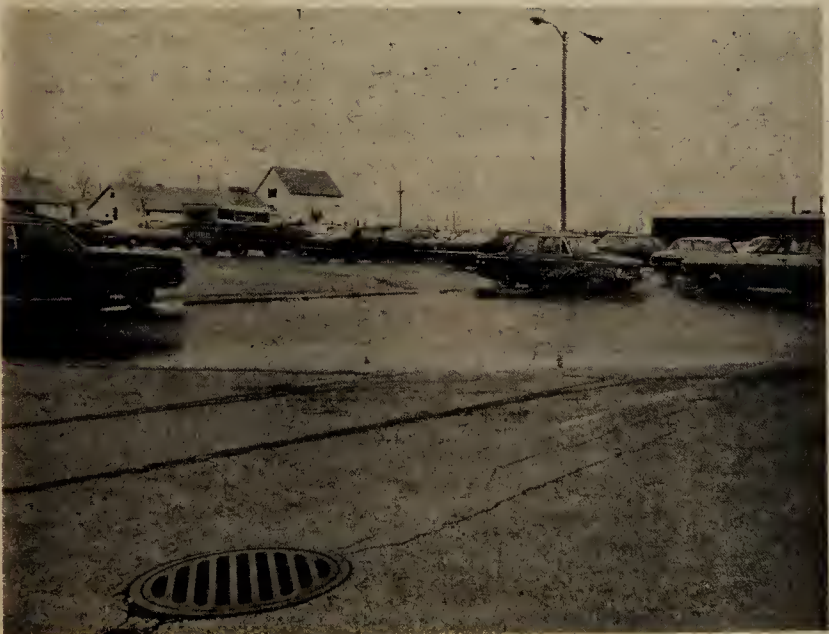
From this picture, you might gather College of DuPage put its drainage on the wrong end of K lot. Not so, says Theodore Zuck, head of Campus Services. The sinkhole developed some two or three years after the drainage pipe was installed. Zuck attributed the sinkhole to boggy ground or a broken section of old farm tile underneath the lot. — Photo by Greg Palumbo.
