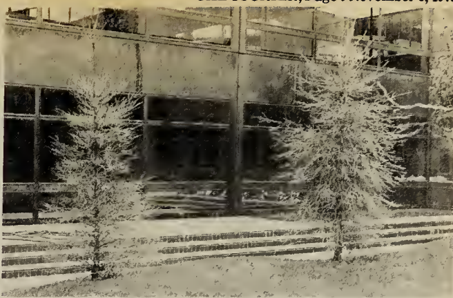
These dead trees near the A Bldg. should be removed soon. They were planted as part of the landscaping project and have since died.
