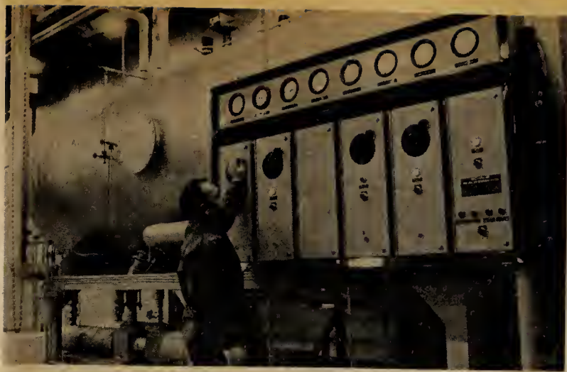
Ken Trout, chief engineer of A Bldg., mans the controls to the boilers in the basement. The heat is distributed throughout the building by four fans and conditions are monitored from different points and relays to a control panel in the boiler room. Photo by Scott Salter.
