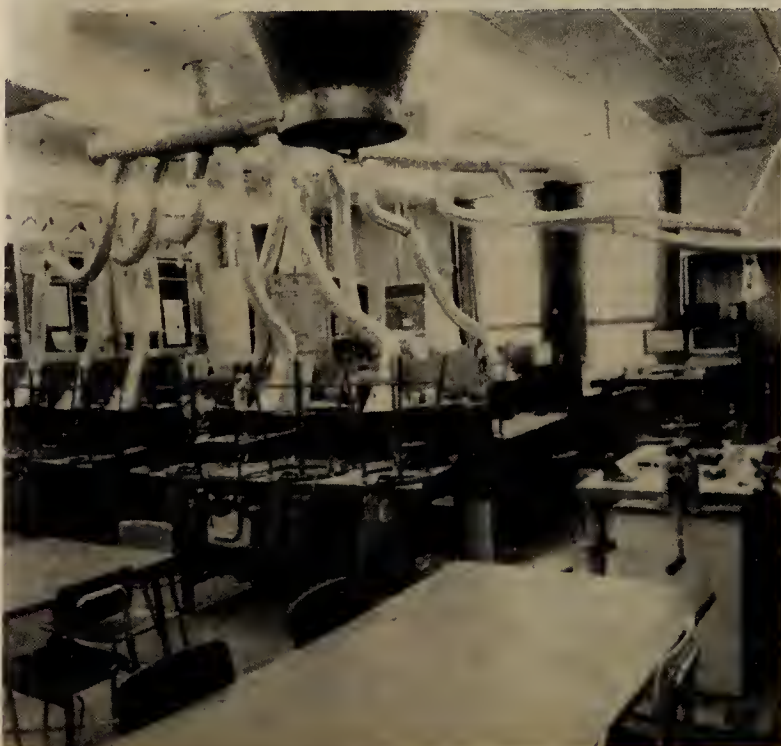
A maze of silvery exhaust tubes dangles from the ceiling in the jewelry lab in M139.
