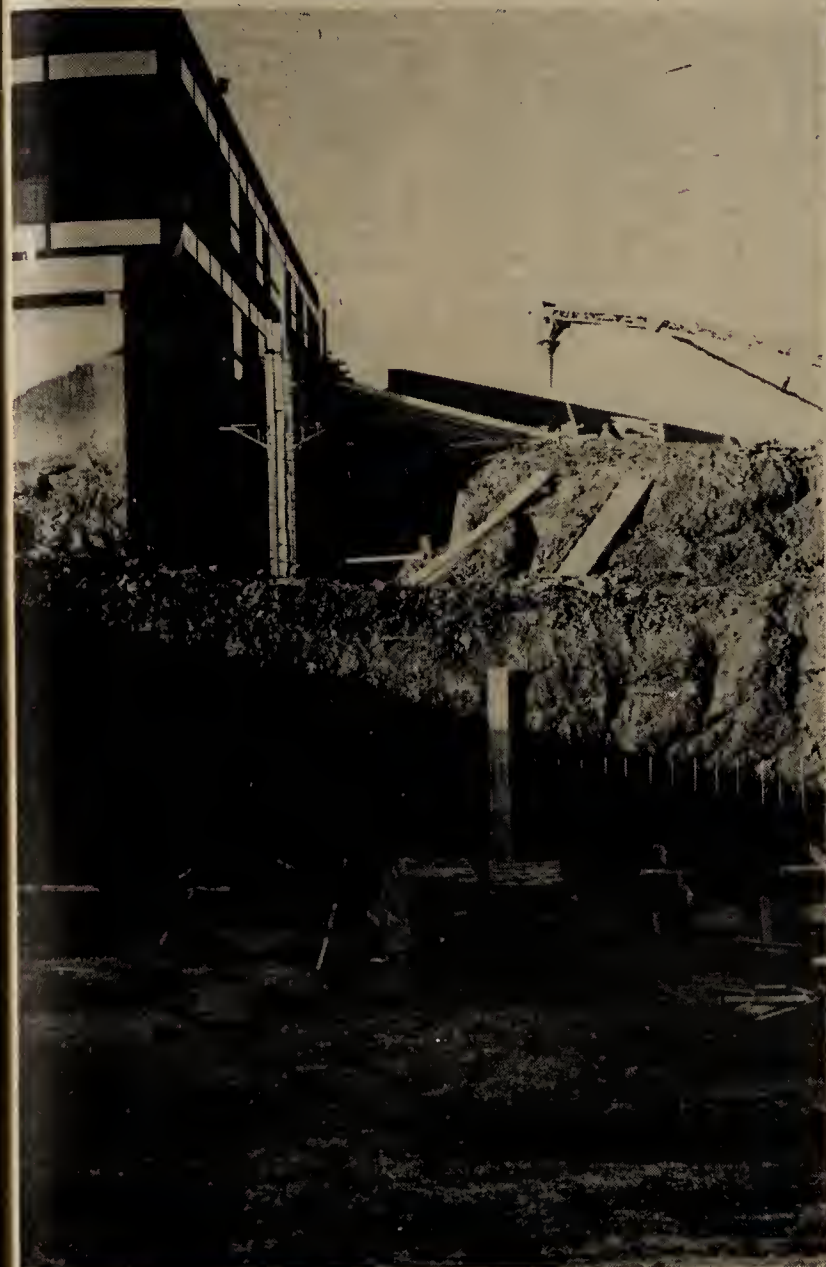
LEFT: EARTH MOVERS CREATED this giant crevice next to Building A. Construction crews excavated soil to depth of 15 feet for foundation of new complex. ABOVE: REINFORCING STEEL RODS jut out above tops of forms for foundation walls in rear as workmen smooth out and inspect freshly poured concrete. BELOW: EAST SIDE OF BUILDING A resembles a moonscape as cement truck prepares to fill wooden forms to cast foundation walls of PE and Community Recreation Center.
