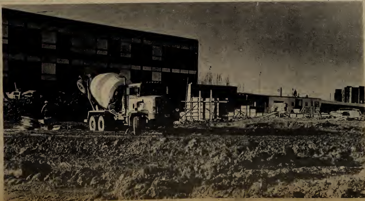
LEFT: EARTH MOVERS CREATED this giant crevice next to Building A. Construction crews excavated soil to depth of 15 feet for foundation of new complex. ABOVE: REINFORCING STEEL RODS jut out above tops of forms for foundation walls in rear as workmen smooth out and inspect freshly poured concrete. BELOW: EAST SIDE OF BUILDING A resembles a moonscape as cement truck prepares to fill wooden forms to cast foundation walls of PE and Community Recreation Center.
