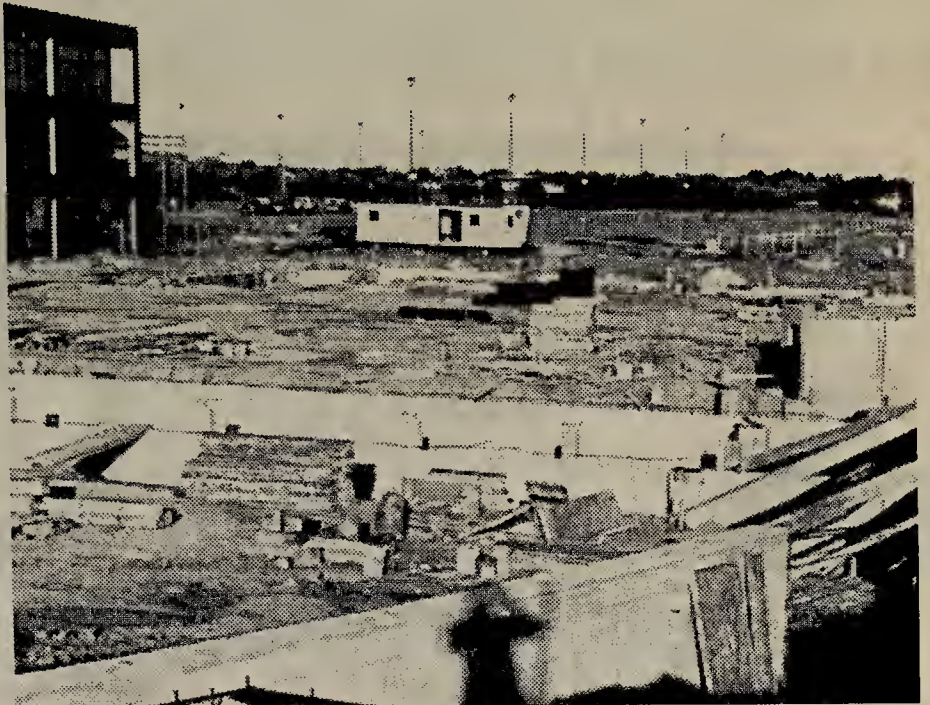
The construction sight as it looked in early July.
